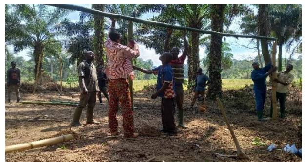
Figure 4: Construction de l'ombrière
