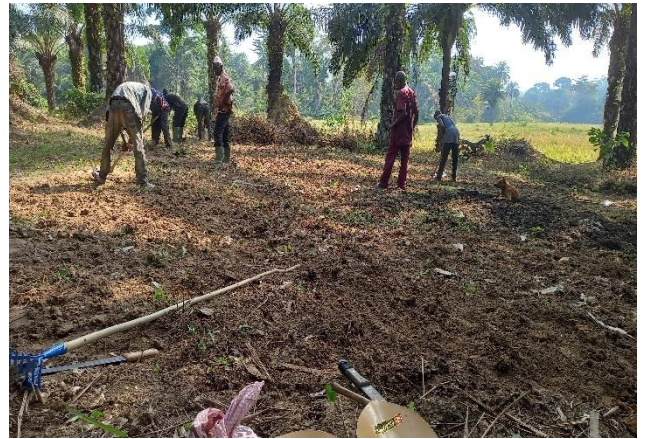
Figure 7: Nettoyage du site
